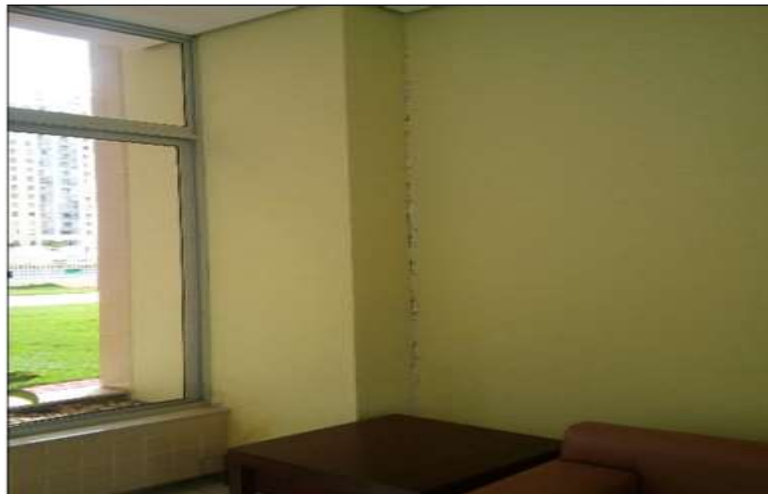
Figura 11 – Trinca Vertical
